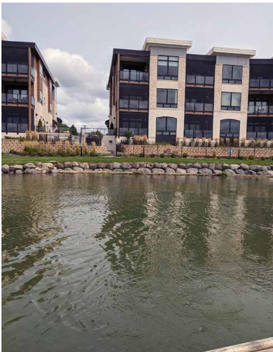
Figure 10. Heavily developed site where a shallow cobble-gravel shoal existed because the riprap was constructed above the high-water level.
