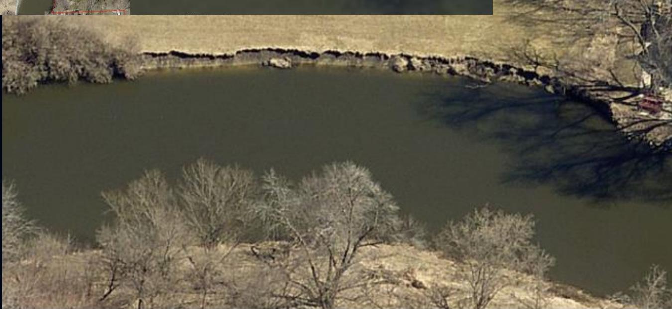
SHOREWOOD TERRACE PARK STREAMBANK STABILIZATION PROJECT 95-4-119-014-1215, Kenosha County
